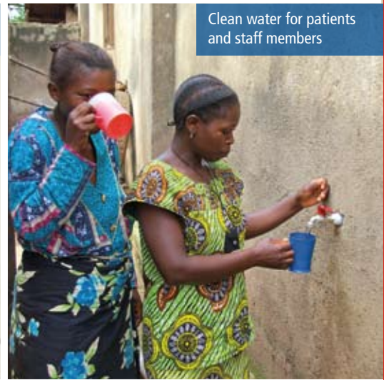
The new water purifier system we installed
